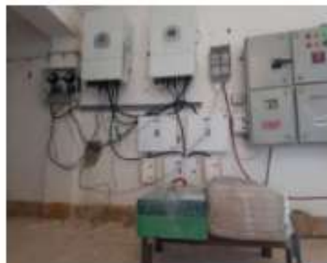
2 X 10KW/D/P Solar Off-Grid System consisting of 100 Ah 48v Solar Batteries and a Solar Hybrid Inverter
